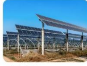
Industrial energy storage
